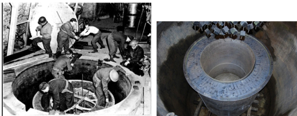
Figure 4. ALSOS team dismantling B-VIII at Haigerloch in 1945 (left) and graphite radial reflector at B-VIII replica at Haigerloch (right), [46]
