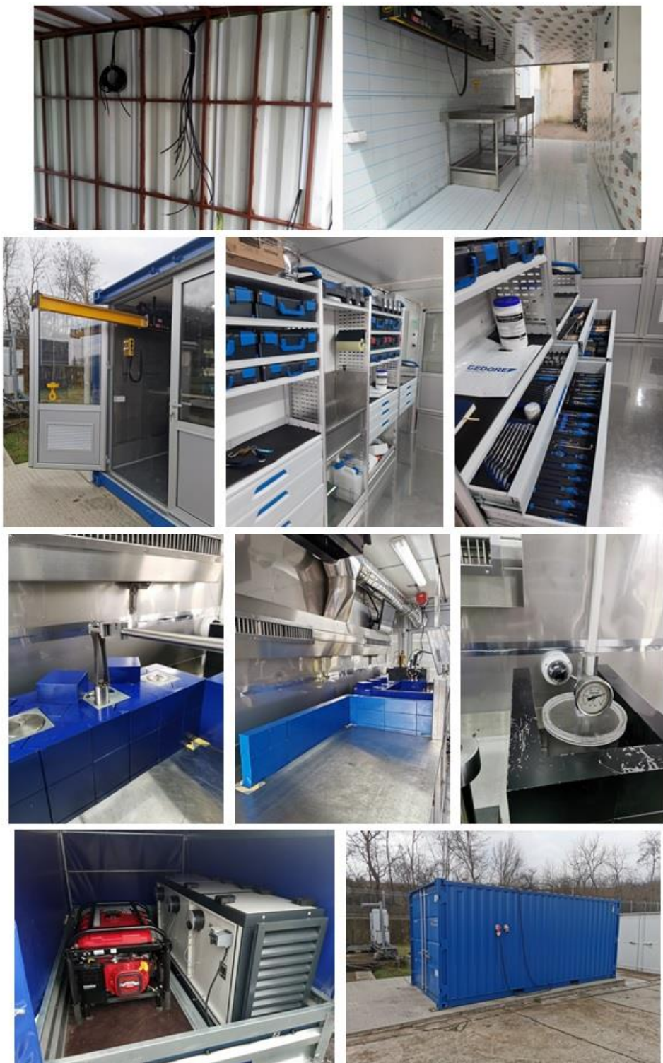
Figure 3. Installation of the MSC DSRs.
