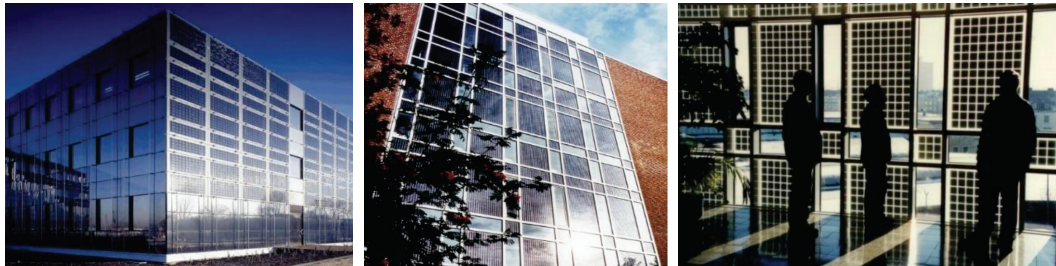
Figure 4. The BIPV façade cladding
