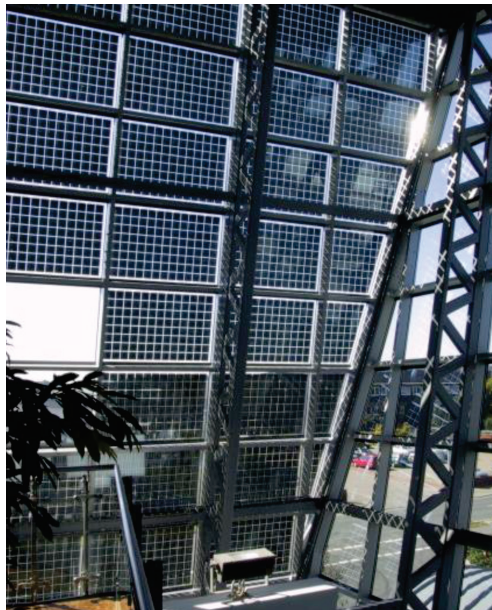
Figure 17. View from exterior of the same façade
