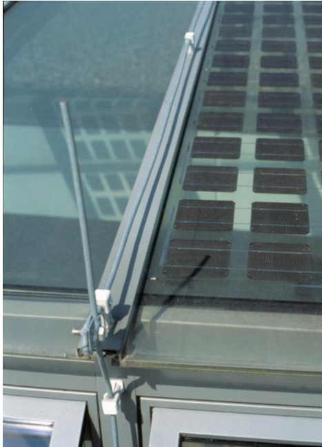
Figure 19. The LPR causing a shadow on the adjacent PV module
