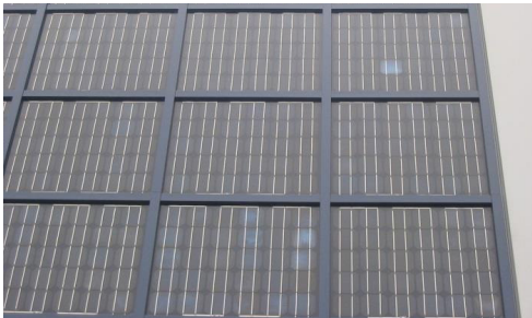
Figure 24. Color variation of PV cells under non-perpendicular examination
