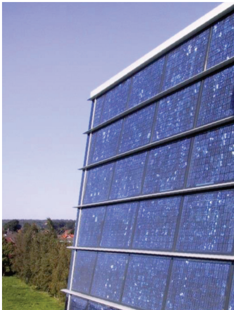
Figure 16. The BIPV façade with cantilevering cover caps to highlight horizontal patterning
