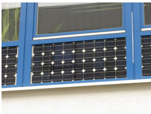
Figure 15. Mezzo-shading caused by a too small distance between solar cell and glass edge
